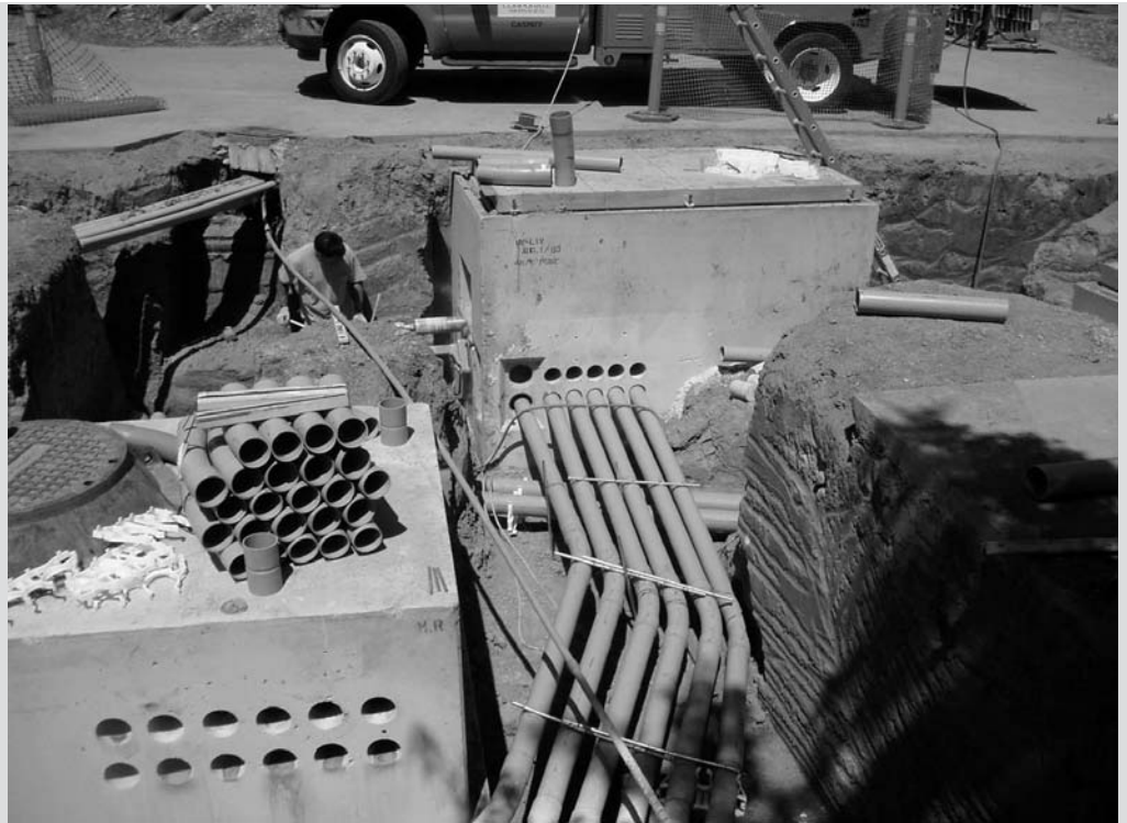
Cabrillo College campus infrastructure improvements
